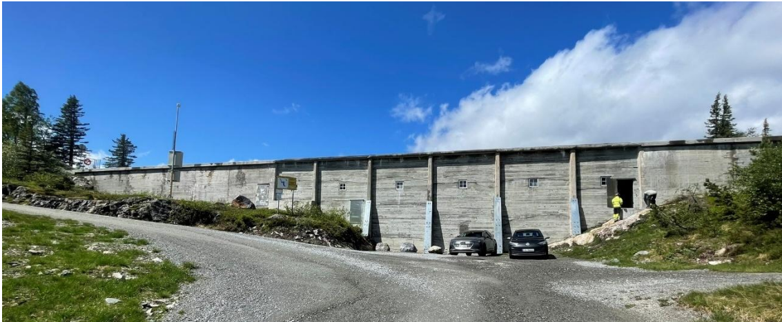
Figure v33. Dam C2, from downstream side. Gravity sections towards each abutment.
