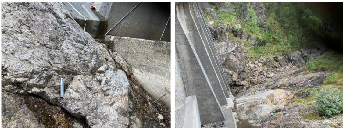
Figure v8. Left: Fractured migmatitic gneiss at bottom of northern valley side, near support E. Right: pegmatitic migmatite undercut by persistent exfoliation joints at middle/upper part of northern valley side.
