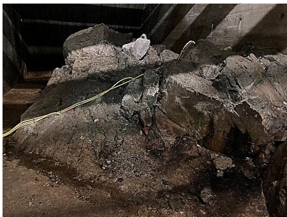
Figure v6. Intermediately fractured, granitic gneiss between support F and G at the bottom of the dam.
