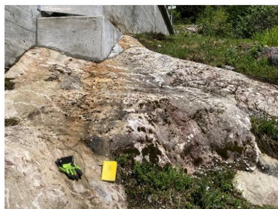
Figure v41: Dam 2: Very massive amphibolite between P7-Ø1 (left) and migmatite at N-end (right).
