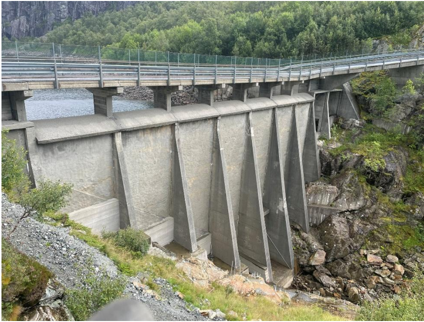
Figure v1. Downstream side of the slab buttress dam. Free overflow spillway along the dam crest.
