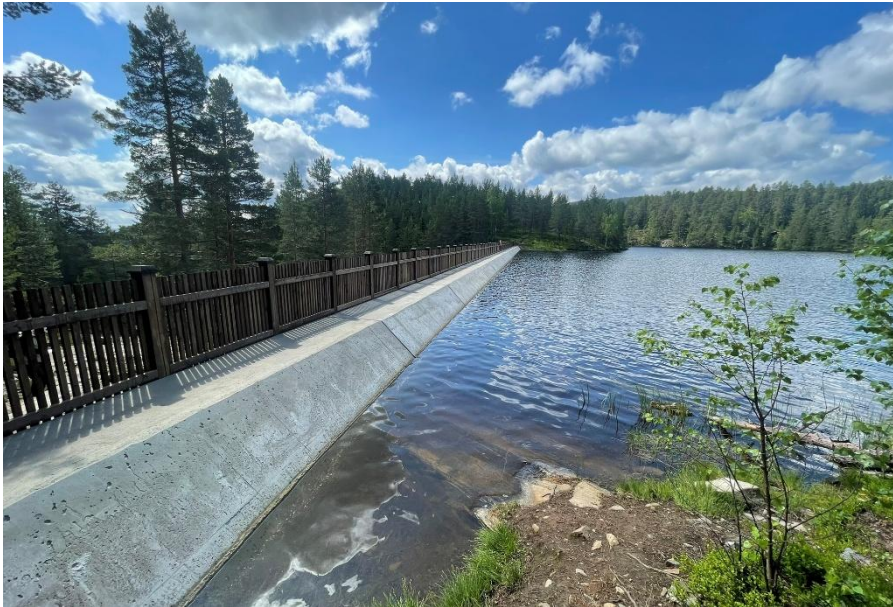
Figure v46. Upstream side with new concrete slab.
