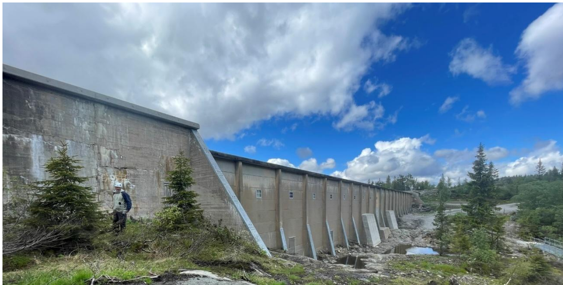
Figure v32. Dam C1, downstream side of the buttress dam, with gravity sections towards each abutment.
