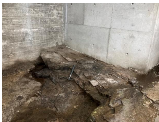
Figure v26: Left: massive syenite with fractures forming tabular blocks at eastern side of dam, P27-28 approx.; Right: more fractured rock at eastern part, P18-19 approx.
