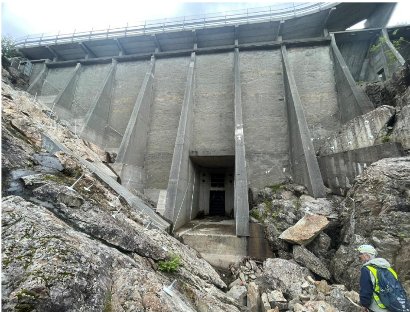
Figure v2. Downstream the bottom gate. Rock bolts and concrete slab to secure the downstream foundation are visible on the downstream foundation.
