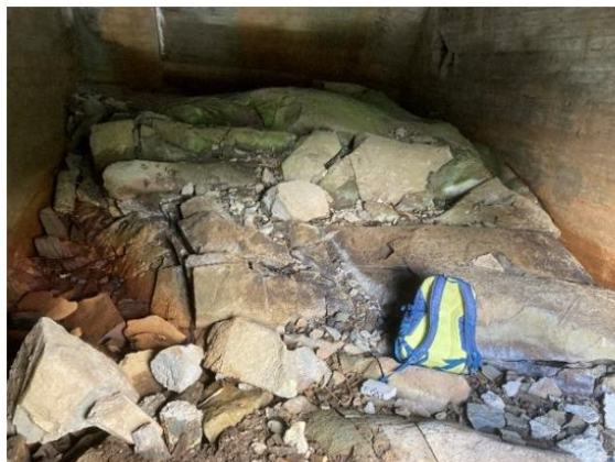
Figure v40: Dam 1: Very massive amphibolite at chamber between support 5 and 6 (left) and mixture of massive and more fractured amphibolite/migmatite at the entrance to hollow section support 5-6 (right).
