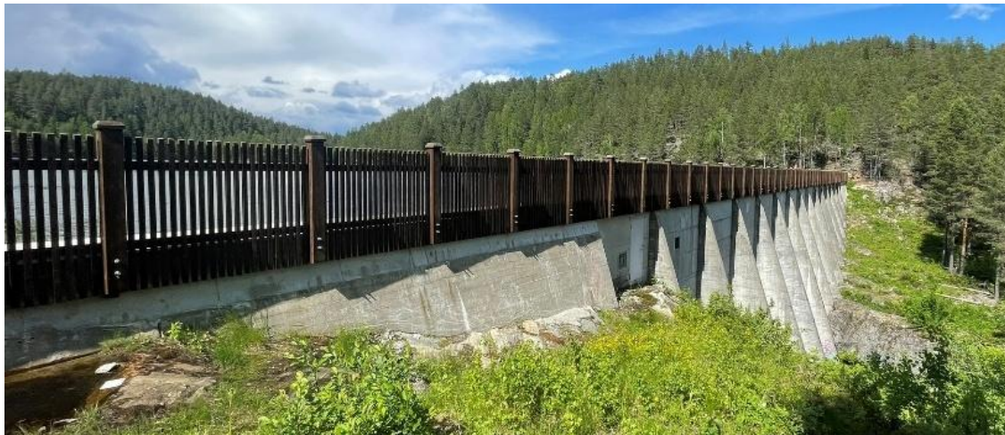
Figure v45. Downstream side of the buttress dam, with gravity sections towards each abutment.
