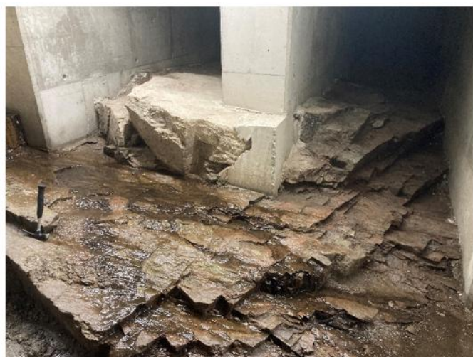
Figure v27. Left: syenite with 3 distinct joint sets, including sub-horizontal, at central part of dam, P16-17 approx. Right: massive syenite at western part of dam, P5-6 approx.
