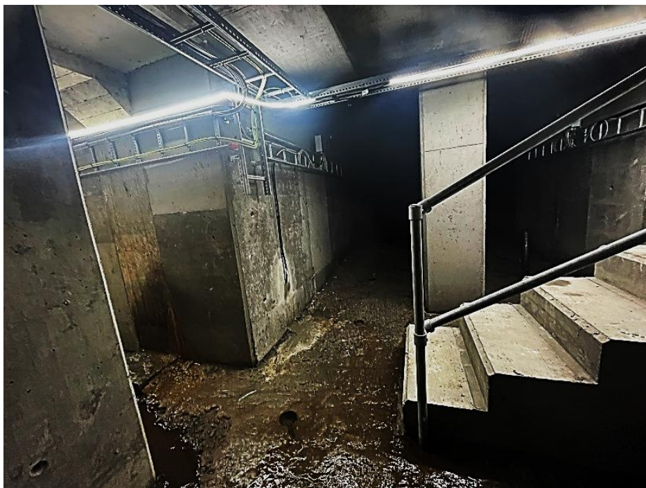
Figure v23. Inspection gallery onto the foundation. View to the upstream side and Buttress supports to the left in the picture.
