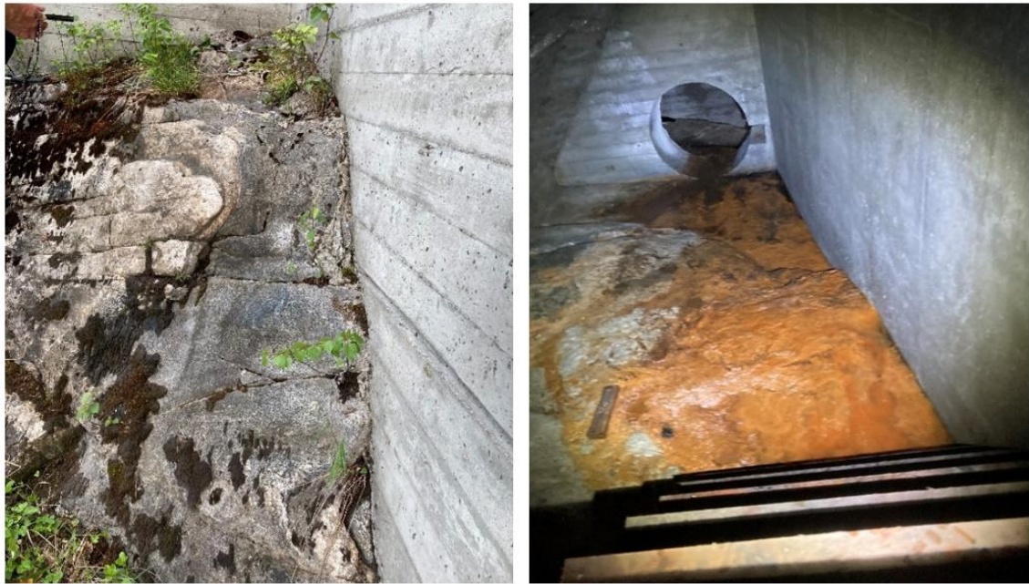
Figure v52. Left: massive rhyolite with distinct planar structure/foliation; Right: water inflow with precipitation of mud-like material from borehole, probably originating from the bottom of the reservoir.
