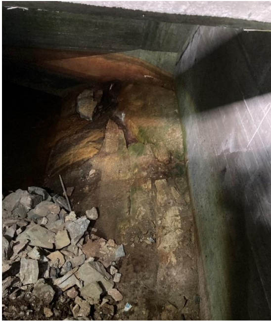
Figure v39: Dam 1: Amphibolite with visible foliation at hollow section between support 3-4.
