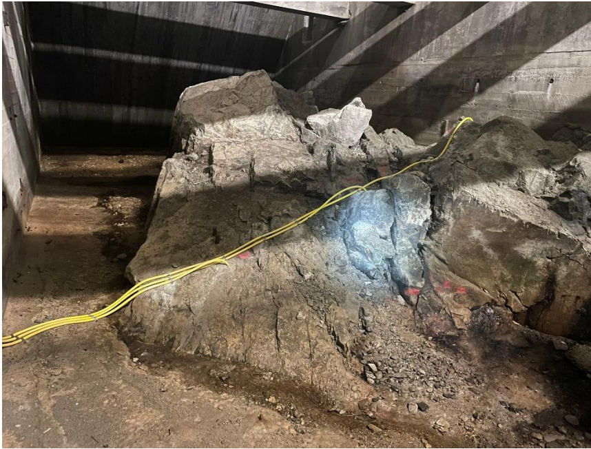
Figure v3. Cables to piezometer P14, P15 and P16.
