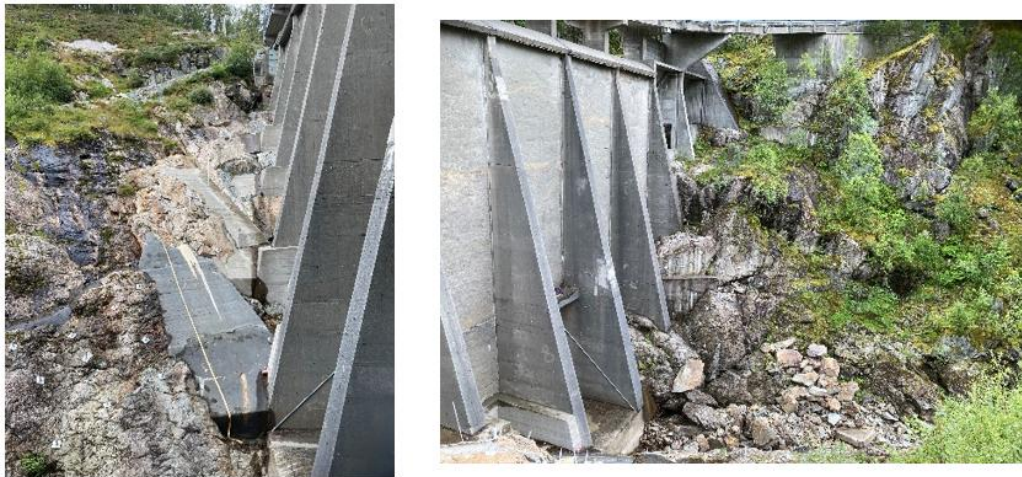
Figure v5: Exposed rock in the downstream slopes of the dam foundation. Left: Migmatitic gneiss at the northern valley side. Mainly massive, but with very distinct exfoliation joints having required heavy rock support. Right: granitic gneiss at the southern valley side, very massive at the middle and upper part, more fractured at lower part.
