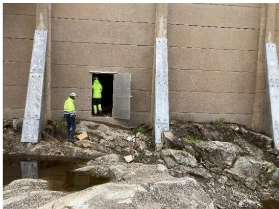
Figure v40: Dam 1: Very massive amphibolite at chamber between support 5 and 6 (left) and mixture of massive and more fractured amphibolite/migmatite at the entrance to hollow section support 5-6 (right).
