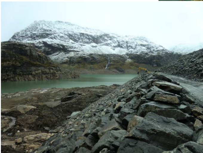
Foto A8, A9, A10 Dam Dravladalen under rehabilitering (2010-2011) (Foto Statkraft)
