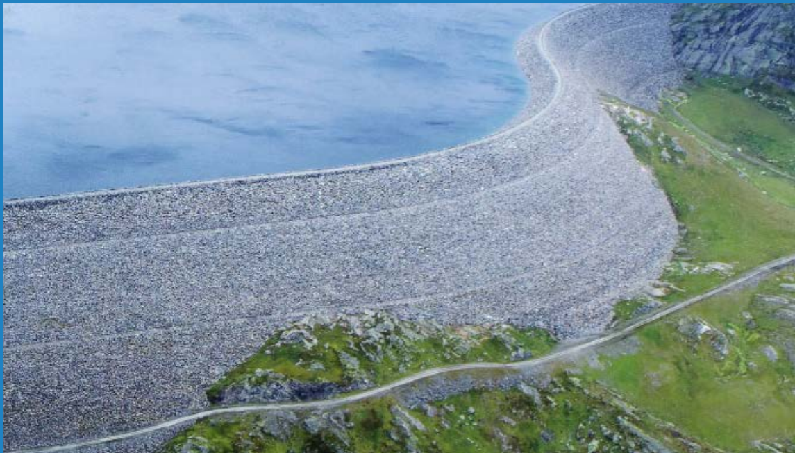
Storvass embankment dam (photo: Statkraft Energi AS)
