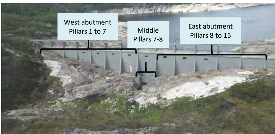
Figure A17. Analysis with FORM and SORM of concrete dam with 15 pillars. Pillar 2 and 5 from the left (west abutment) were the most critical
