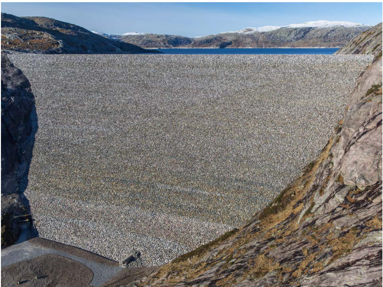
Svartevatn Dam (Photo: Sira Kvina)
