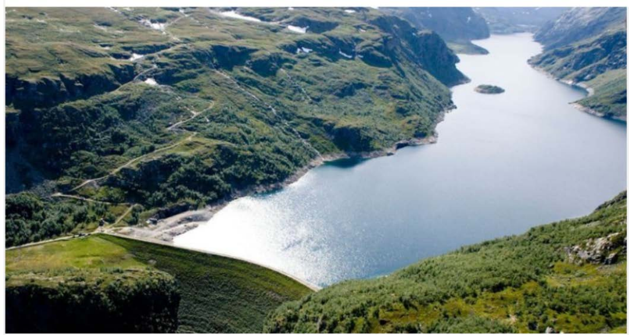
Viddalsvatn Dam in Aurland County (Photo Hafslund Eco)
