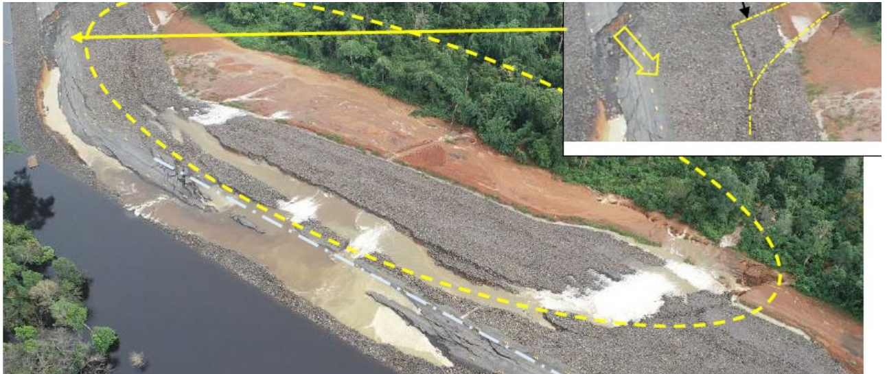
Figure 48: Overview of the dam failure of Xe-Pian saddle dam D [21].
