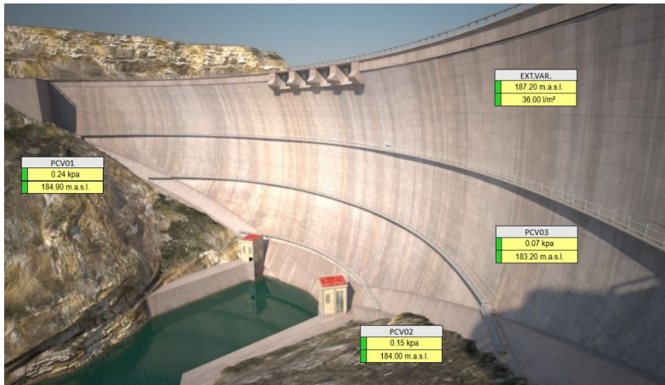
Figure 28: Visualization of real time values and alarm levels over 3D model of a dam.
