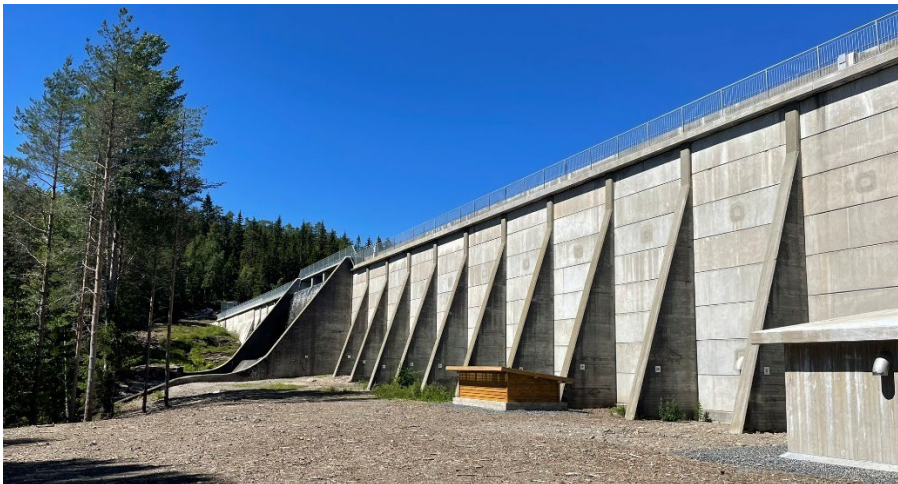
Figure v22. Downstream side of the buttress dam. The original frost wall and buttress supports are visible from the downstream side. However, upstream the frost wall the whole dam has been filled with concrete, except the lower part over the foundation, where there is an inspection gallery.
