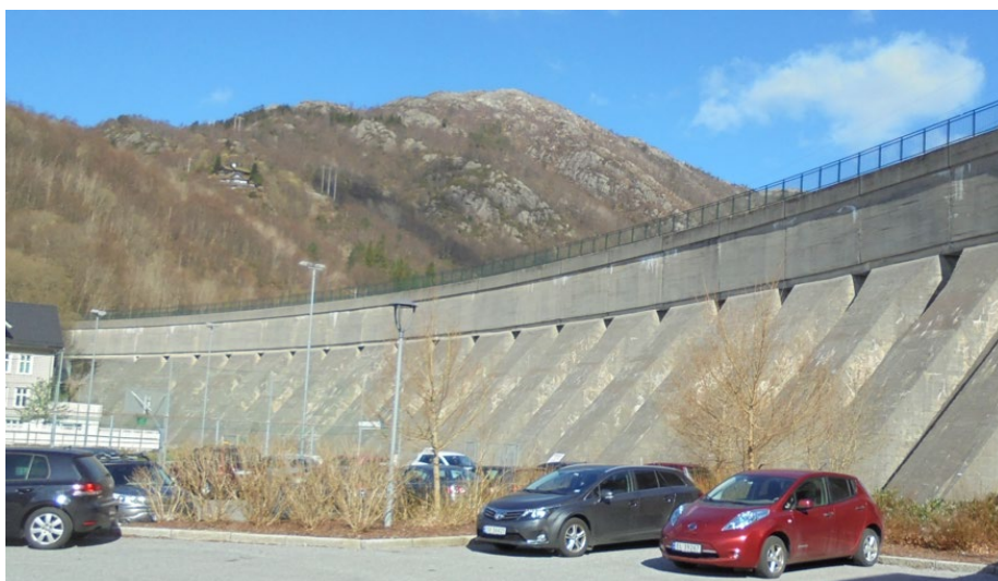
Figur 5 Lamelldam, Dam Svartediket (photo: T.Konow).
