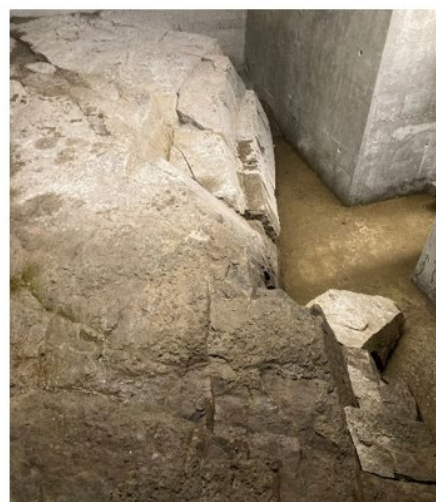
Figure v27. Left: syenite with 3 distinct joint sets, including sub-horizontal, at central part of dam, P16-17 approx. Right: massive syenite at western part of dam, P5-6 approx.
