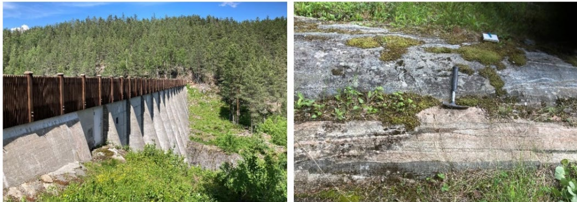
Figure v51: Left: overview of the dam as seen from south; Right: very massive bedrock with distinct banding near the northern end
