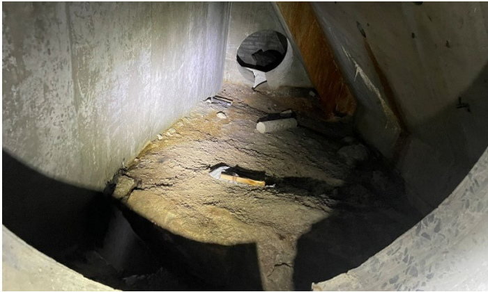
Figure 110. Drainage gallery in front of buttress.
