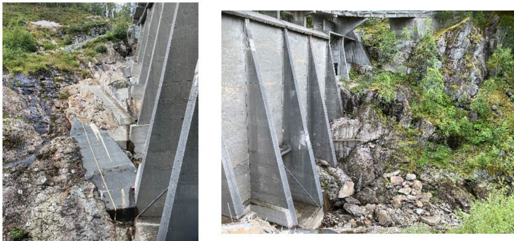
Figure 67: Exposed rock in the downstream slopes of the dam foundation. Left: Migmatitic gneiss at the northern valley side. Mainly massive, but with very distinct exfoliation joints having required heavy rock support. Right: granitic gneiss at the southern valley side, very massive at the middle and upper part, more fractured at lower part.
