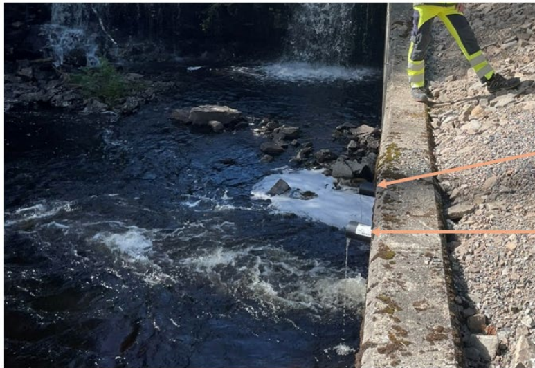
Figure 87. Drains with leakage. One pipe from each side of the dam
