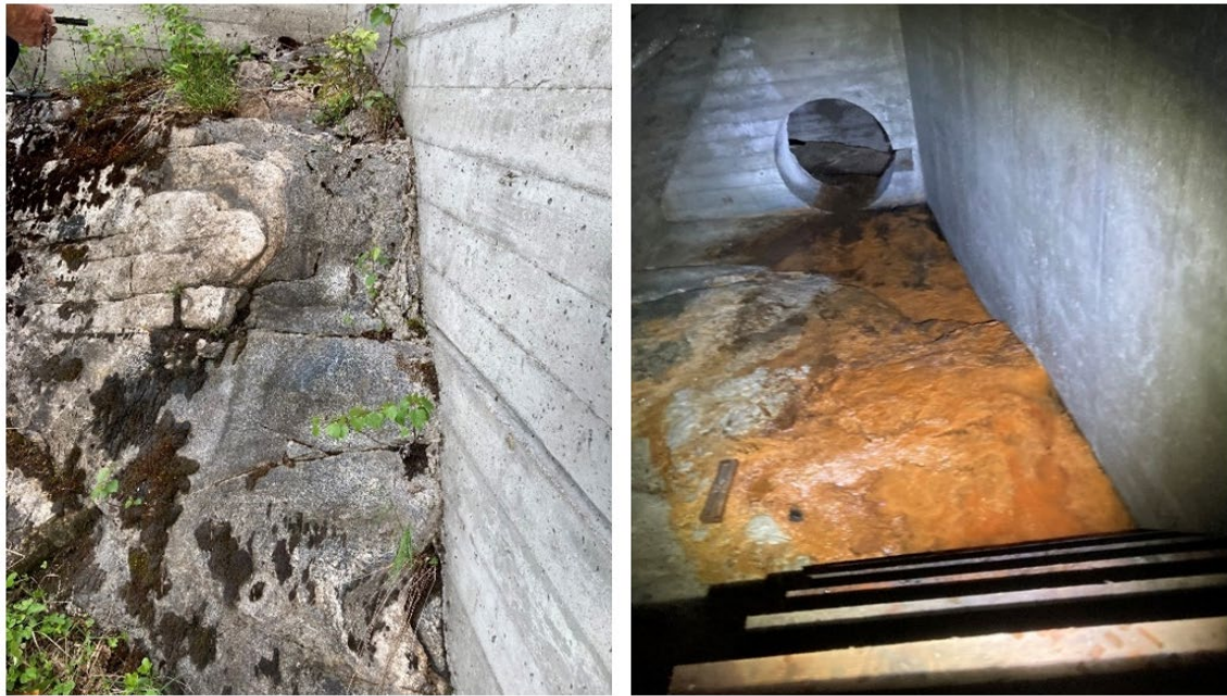
Figure 114. Left: massive rhyolite with distinct planar structure/foliation; Right: water inflow with precipitation of mud-like material from borehole, probably originating from the bottom of the reservoir.
