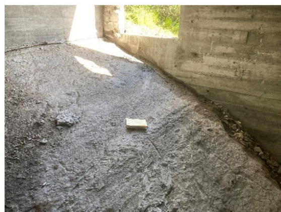
Figure 103. Dam 2: Very massive amphibolite between P7-Ø1 (left) and migmatite at N-end (right).
