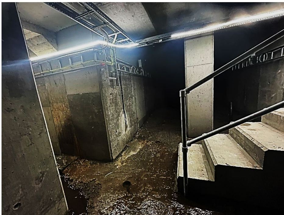
Figure 85. Inspection gallery onto the foundation. View to the upstream side and Buttress supports to the left in the picture.
