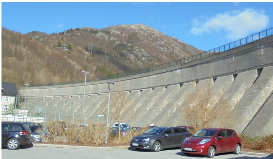
Figure 5. Solid head buttress dam, Dam Svartediket (photo: T.Konow).
