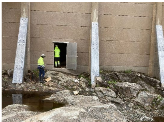
Figure 102. Dam 1: Very massive amphibolite at chamber between support 5 and 6 (left) and mixture of massive and more fractured amphibolite/migmatite at the entrance to hollow section support 5-6 (right).
