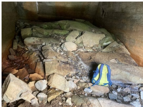
Figure 102. Dam 1: Very massive amphibolite at chamber between support 5 and 6 (left) and mixture of massive and more fractured amphibolite/migmatite at the entrance to hollow section support 5-6 (right).
