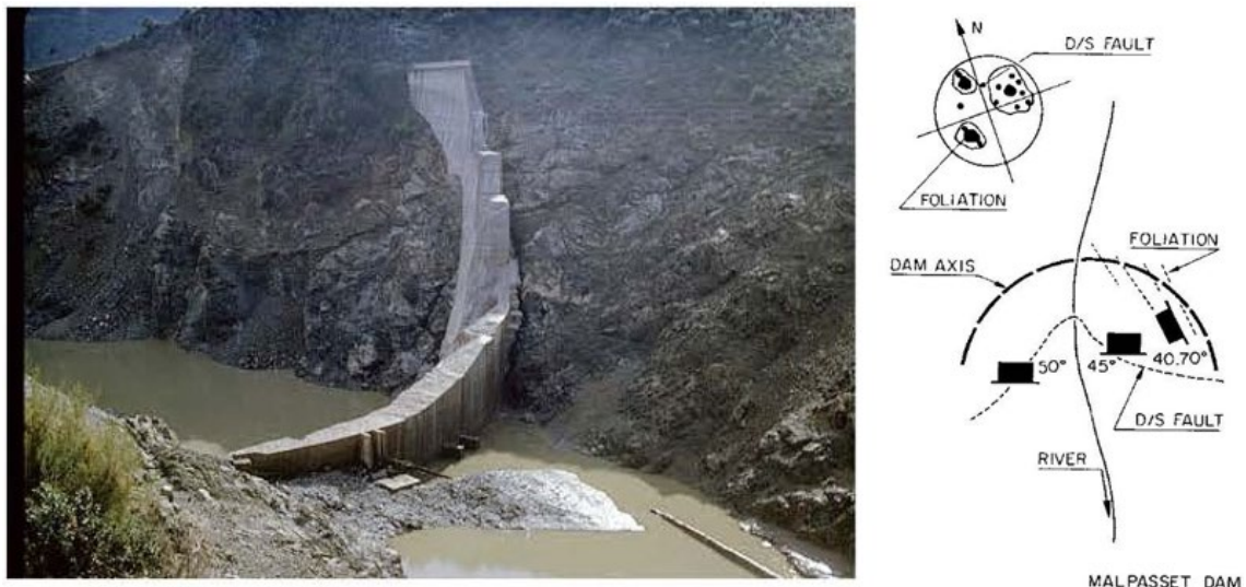
Figure 43: Failure of left abutment of Malpasset dam due to unfavourably oriented fault dipping 45-50° upstream and foliation fractures dipping 40°W (plot in stereographic projection, upper hemisphere). Left photo from (Duffault, 2012), sketch to the right from (Goodman, 1993).
