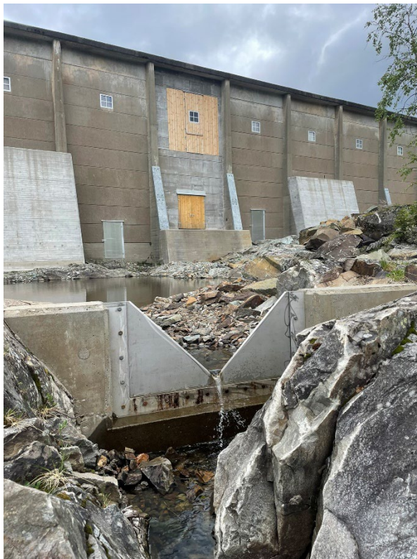
Figure 99. Dam C1 - leakage from the dam with full reservoir, about 0.1 l/s.
