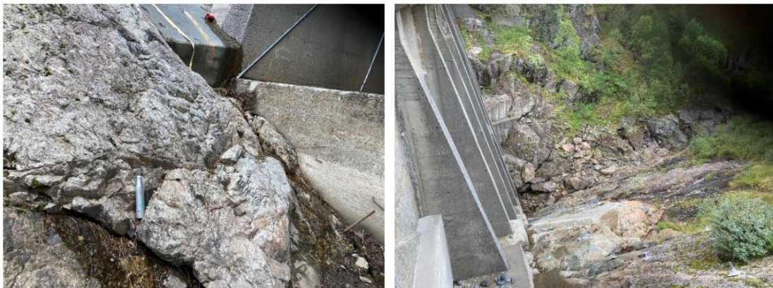
Figure 70. Left: Fractured migmatitic gneiss at bottom of northern valley side, near support E. Right: pegmatitic migmatite undercut by persistent exfoliation joints at middle/upper part of northern valley side.
