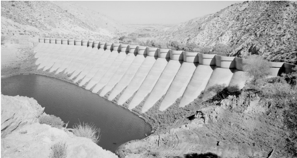
Figure 6. Buttress dam: Upstream side of a multiple arch dam (Photo: National Park Service, US)
