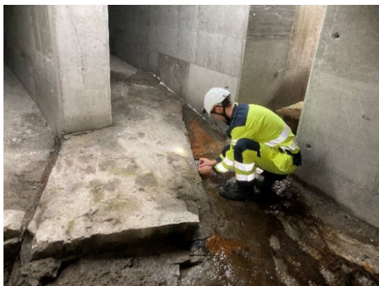
Figure 88: Left: massive syenite with fractures forming tabular blocks at eastern side of dam, P27-28 approx.; Right: more fractured rock at eastern part, P18-19 approx.
