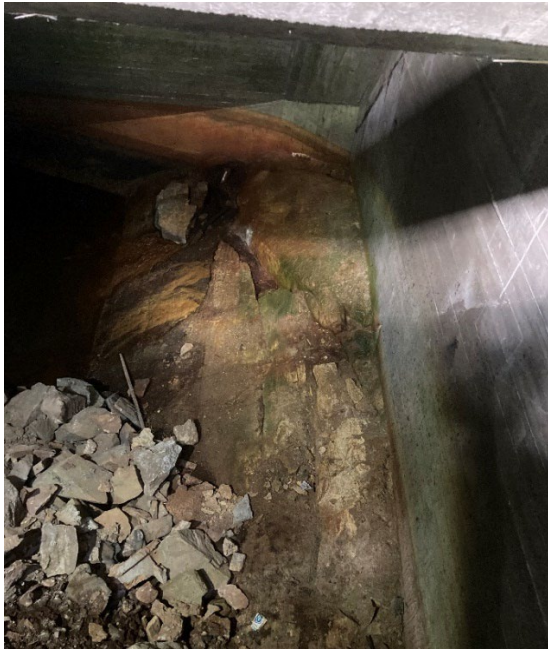
Figure 101: Dam 1: Amphibolite with visible foliation at hollow section between support 3-4.
