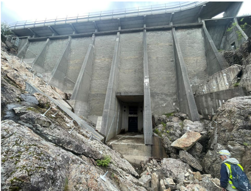
Figure 64. Downstream the bottom gate. Rock bolts and concrete slab to secure the downstream foundation are visible on the downstream foundation.
