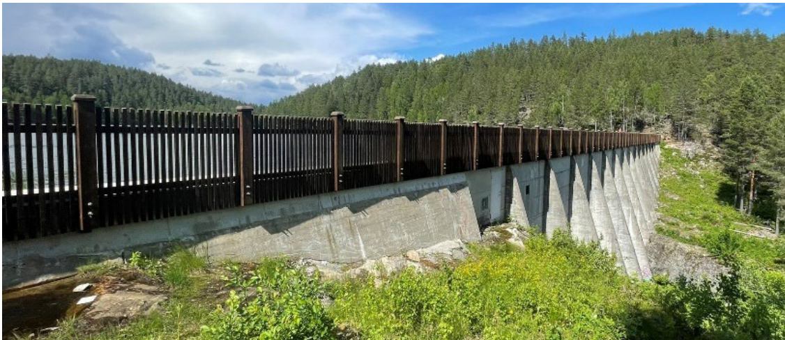
Figure 107. Downstream side of the buttress dam, with gravity sections towards each abutment.
