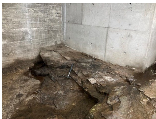
Figure 88: Left: massive syenite with fractures forming tabular blocks at eastern side of dam, P27-28 approx.; Right: more fractured rock at eastern part, P18-19 approx.
