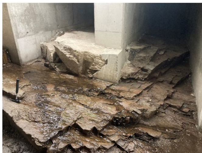
Figure 89: Left: syenite with 3 distinct joint sets, including sub-horizontal, at central part of dam, P16-17 approx. Right: massive syenite at western part of dam, P5-6 approx.
