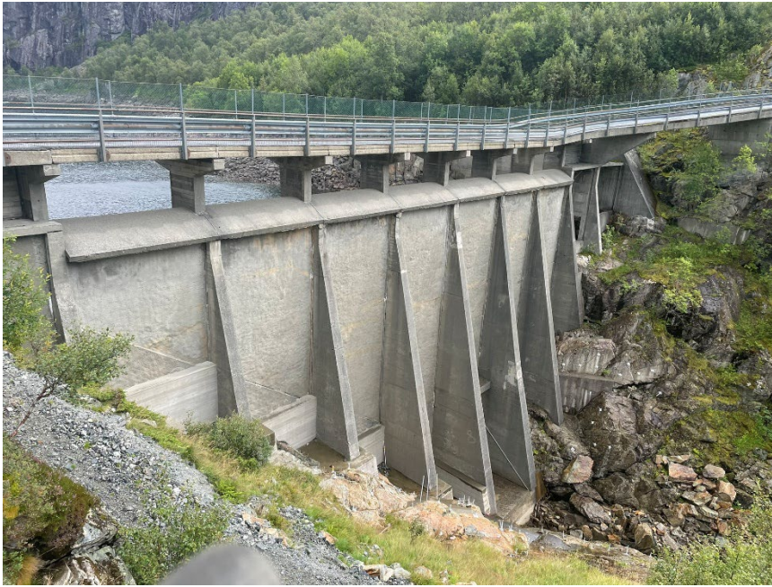
Figure 63. Downstream side of the slab buttress dam. Free overflow spillway along the dam crest.
