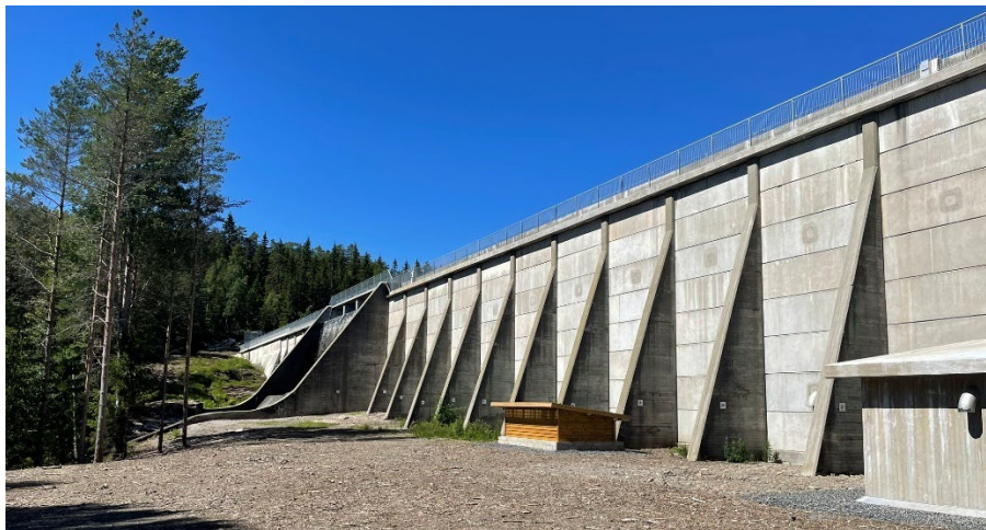
Figure 84. Downstream side of the buttress dam. The original frost wall and buttress supports are visible from the downstream side. However, upstream the frost wall the whole dam has been filled with concrete, except the lower part over the foundation, where there is an inspection gallery.
