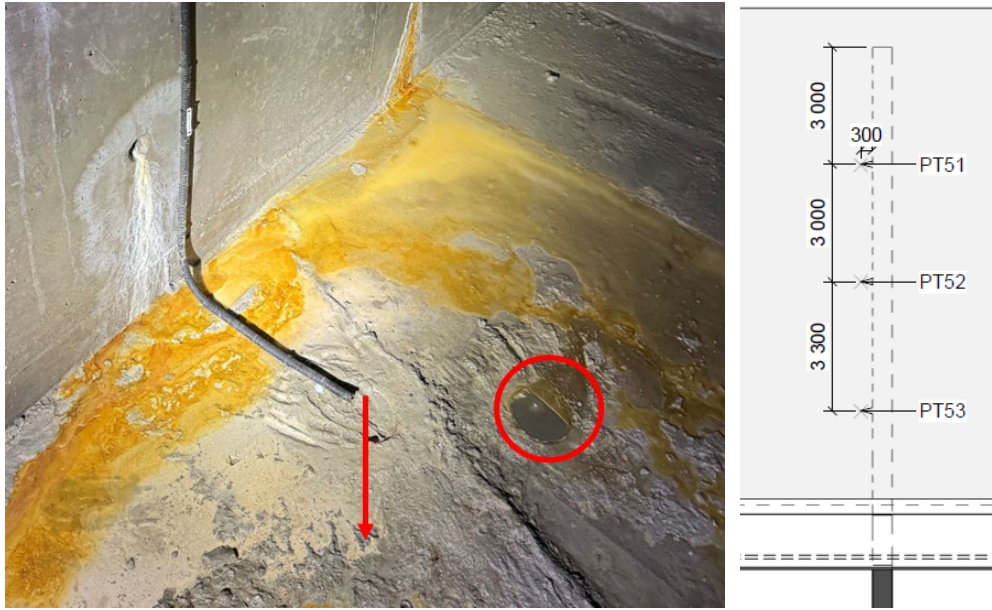
Figure 93 Picture of sensor and bore hole location/Cutout from drawings
