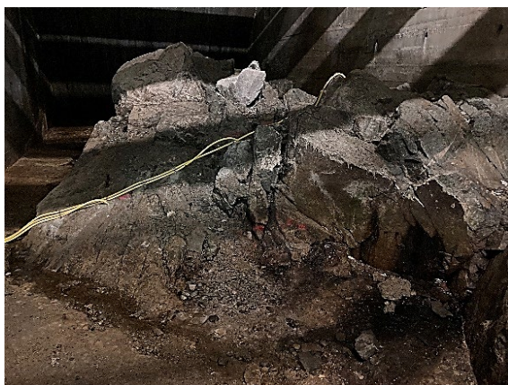
Figure 68. Intermediately fractured, granitic gneiss between support F and G at the bottom of the dam.
