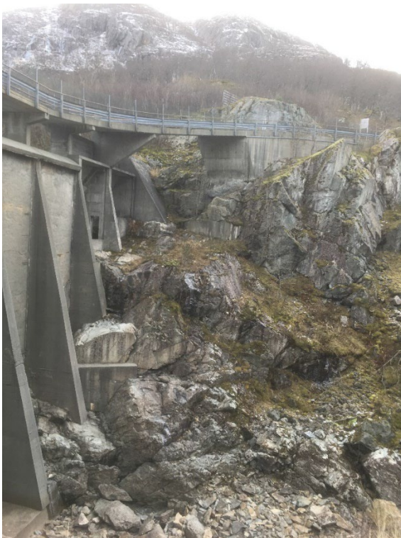
Figure 44: Example illustrating fracturing with varying orientation and persistence at dam abutment.
