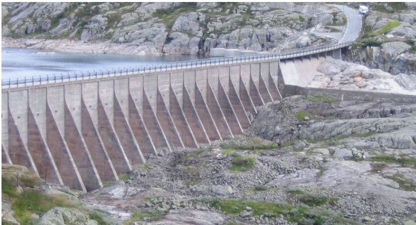
Figure 7. Slab buttress dam. Dam Svartevatn (photo: NVE/Karen Marie Straume)
