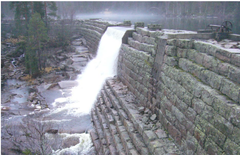
Figure 3. Dry laid masonry dam(photo. T.Konow)
