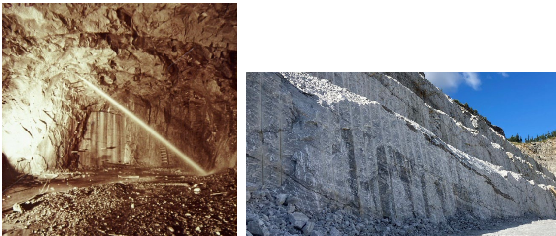
Figure 42: Left : Concentrated flow-pipe/channel in fracture intersecting deep tunnel (Kvittdal HPP, from NTNU slide-archive), Right: Water leakage from very continuous joint at face of long rock slope; leakage is not evenly distributed, but concentrated to certain sections/flow channels (photo B. Nilsen).
