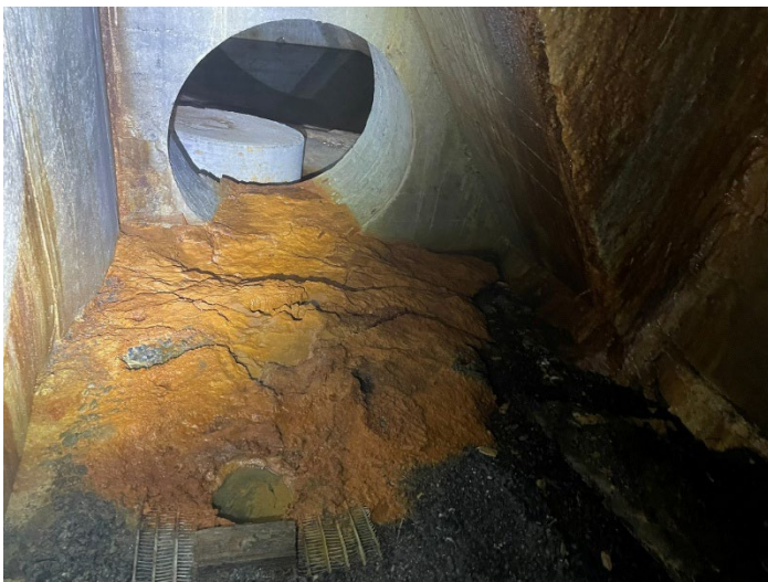
Figure 111. Some of the drains have water seepage with mud-like material from borehole.
