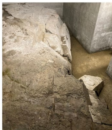
Figure 89: Left: syenite with 3 distinct joint sets, including sub-horizontal, at central part of dam, P16-17 approx. Right: massive syenite at western part of dam, P5-6 approx.
